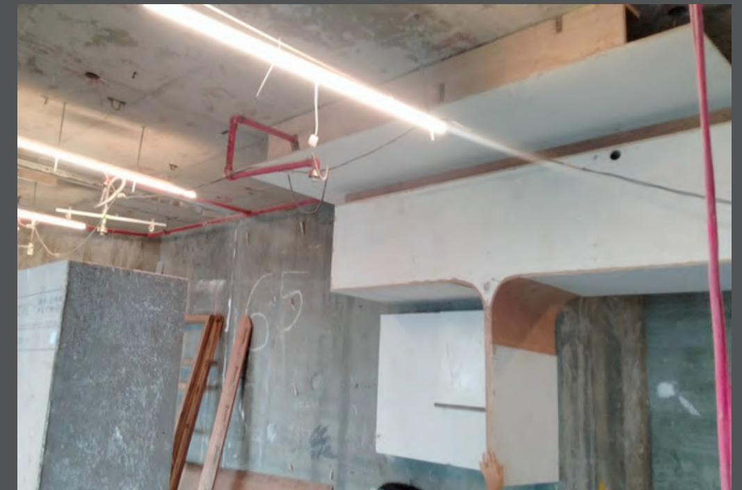
CEILING MOCK UP
